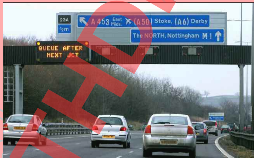
Figure 5. Portal gantry mounted 2 x 12 Message Sign.
