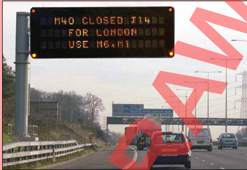
Figure 3. 3 x 18 Motorway Signal Mark 3 (MS3) - the MS4 is not an alternative to this MS3.
