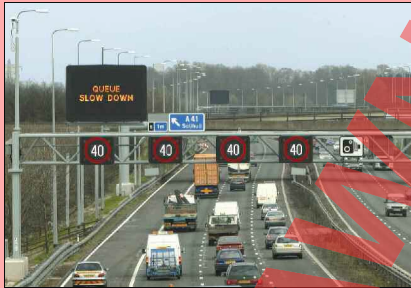
Figure 4. MS4 display panel mounted on a portal gantry as part of the ATM Pilot being used as a Message Sign. Panel size 4.44m by 3.16m
