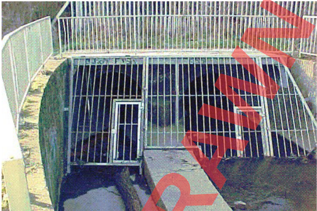
Plate A5: Example of a Screen to a Large Watercourse
