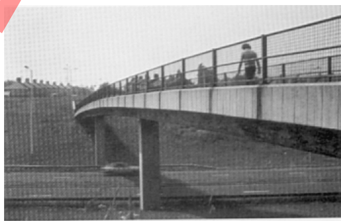
Figure 15. Streaking due to a mistake in detailing. The top of the fascia/parapet plinth was detailed without an inward fall. Correctly detailed bridges with similar parapets on the same contract are not streaked.
