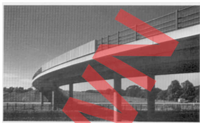
Figure 12. Treatment of a high containment parapet to emphasise the continuity of the deck. A step in the face of the parapet to create a shadow line, and a different surface, which should not be overdone.
