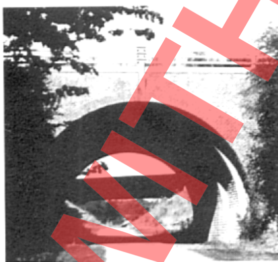
20a & b. The bridge designed by Sir Edwin Lutyens to take the A3 over the Pilgrim's Way near Compton in Surrey, seen in relation to a more modern bridge which carries the realigned A3. Notice how Lutyens has used the device of stepping the arch at each end of the tunnel, to increase the apparent size of the arch in elevation and to reduce the tunnel effect.
