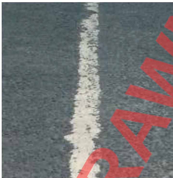
Figure E9: Condition Score 20 – close-up of profiled line designed for wet visibility
