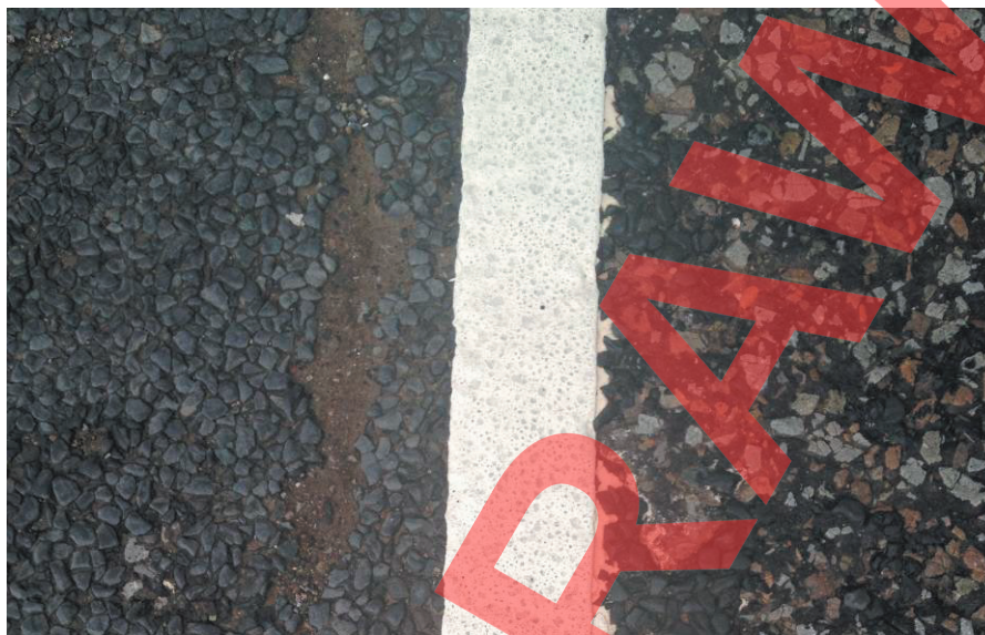
Figure E2: Condition Score 50 – close-up of profiled line designed for wet visibility
