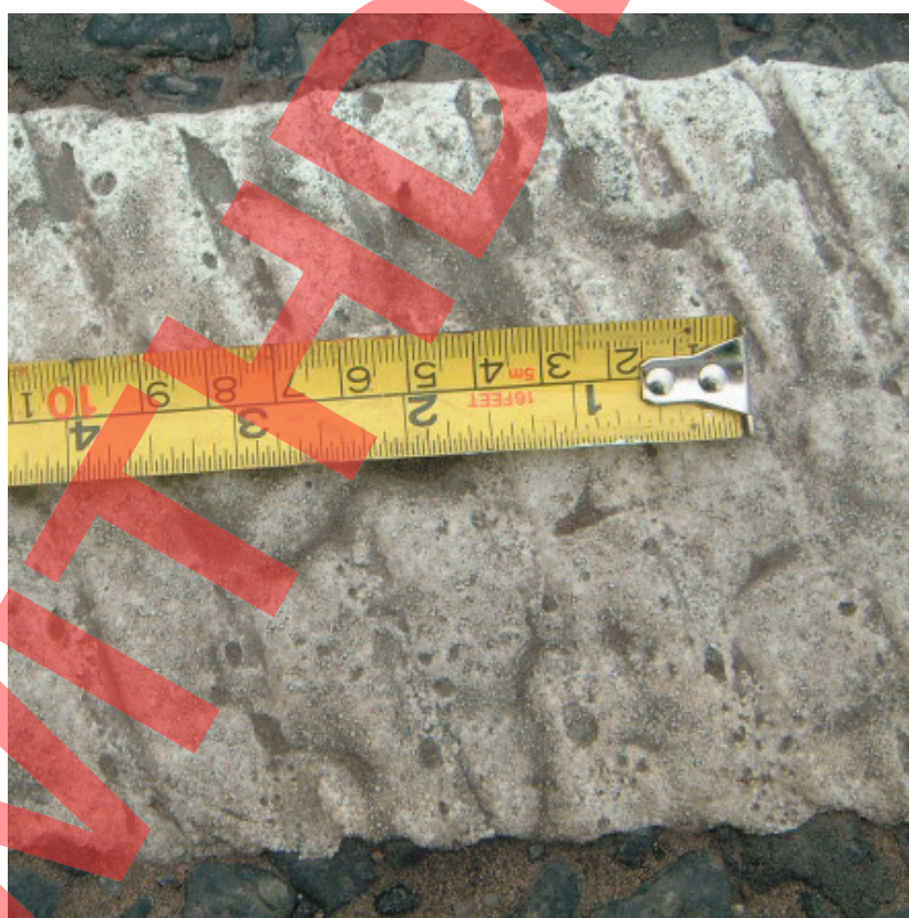
Figure E9: Condition Score 20 – close-up of profiled line designed for wet visibility
