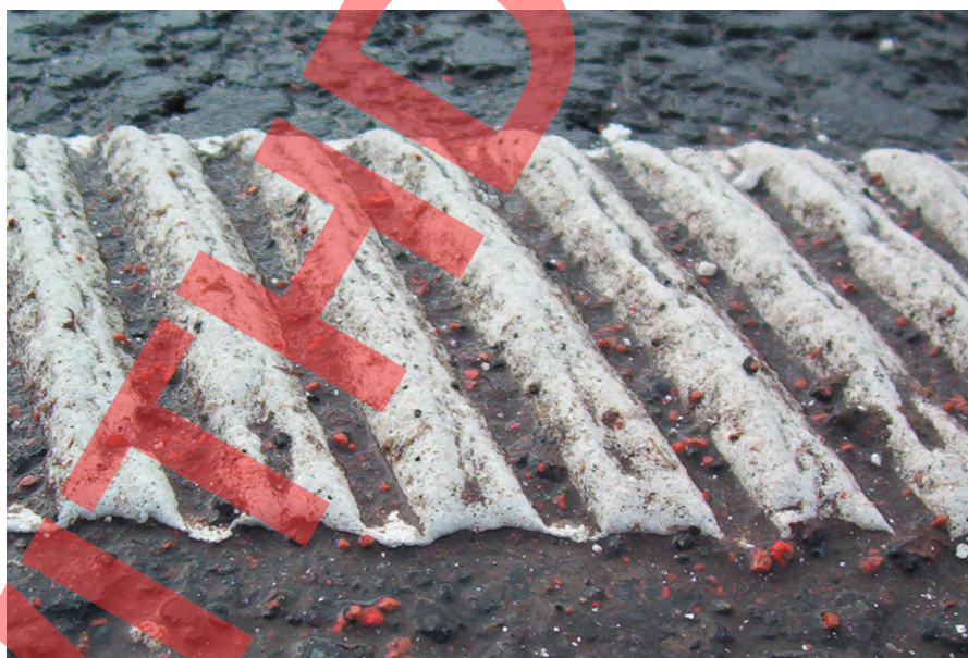
Figure E2: Condition Score 50 – close-up of profiled line designed for wet visibility
