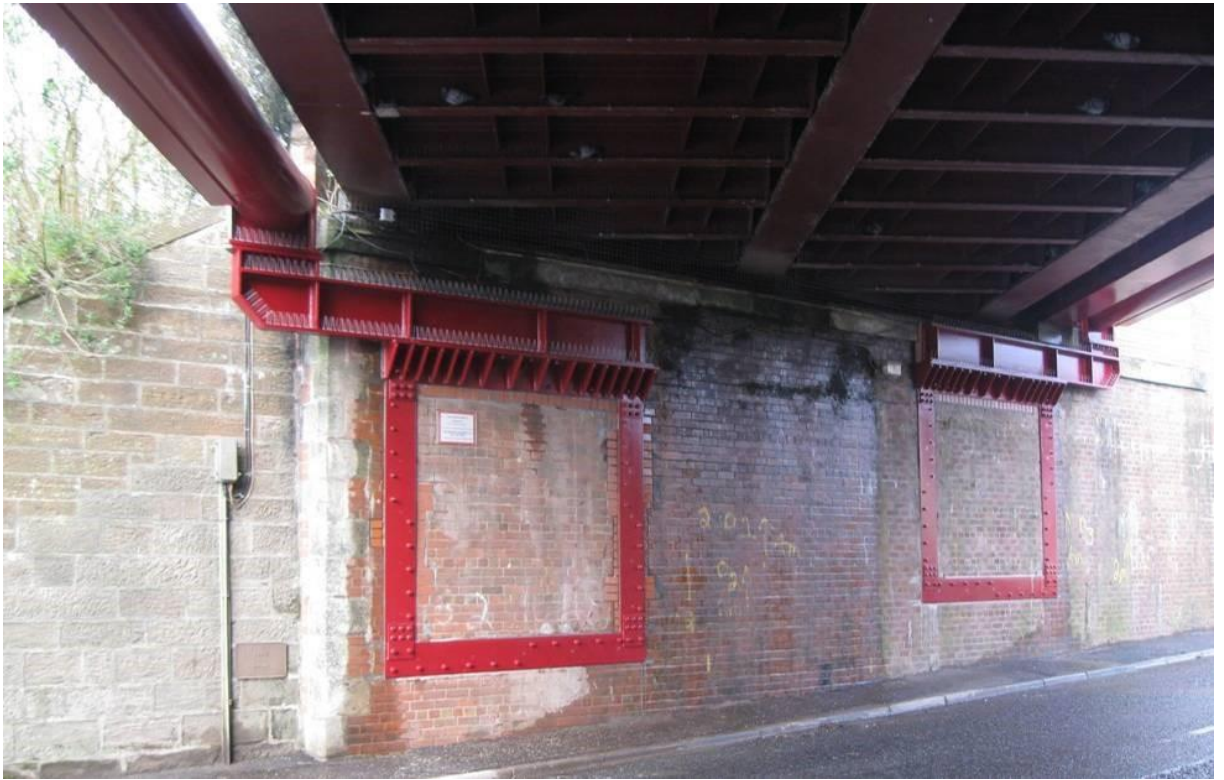
Figure A.2 Collision protection beam abutment supports
