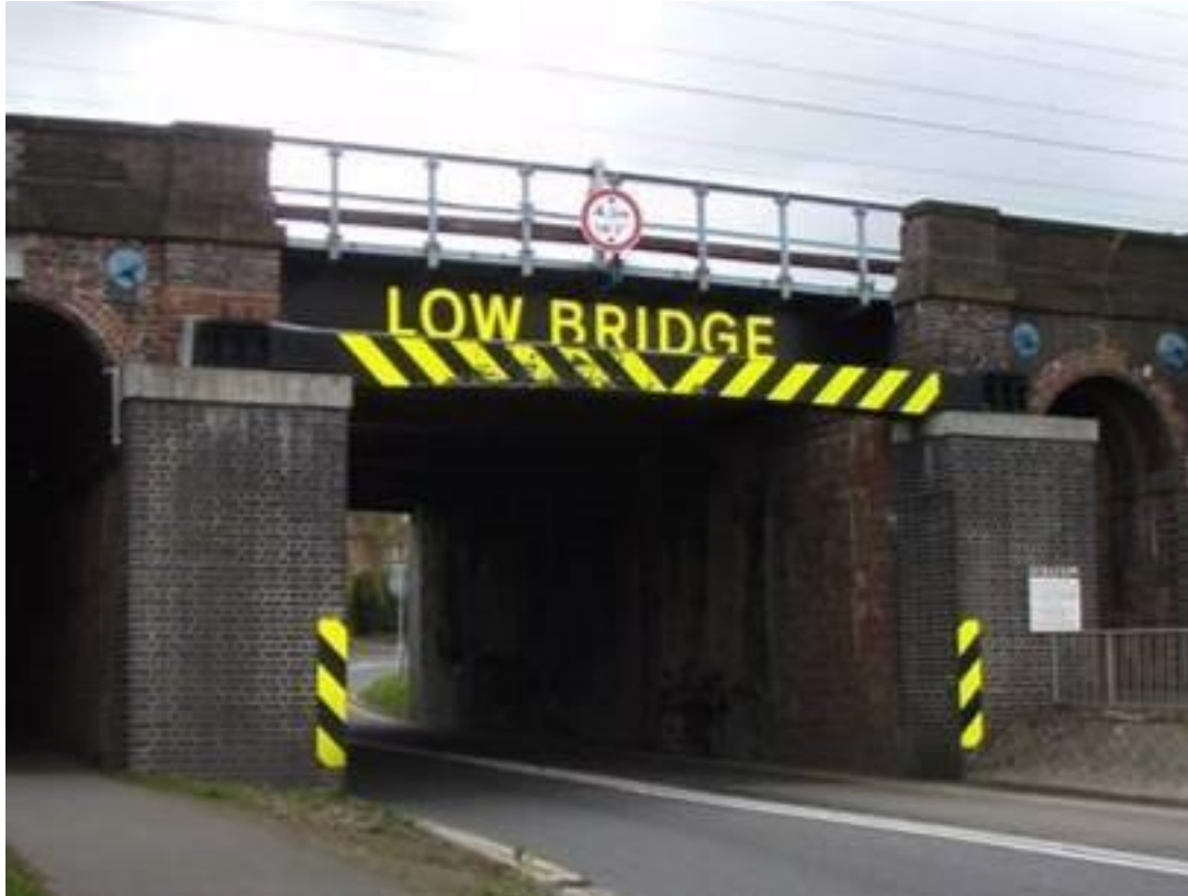
Figure A.6 Collision protection beam to flat soffit bridge supported from abutment extensions. Note the camber to the beam
