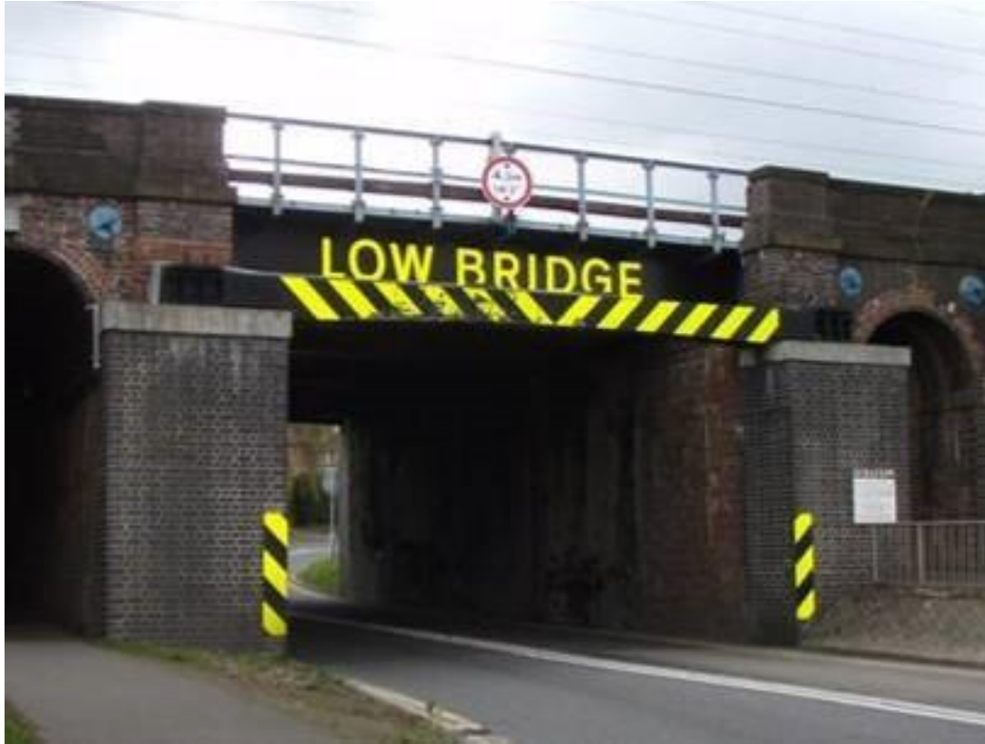
Figure A.6 Collision protection beam to flat soffit bridge supported from abutment extensions. Note the camber to the beam
