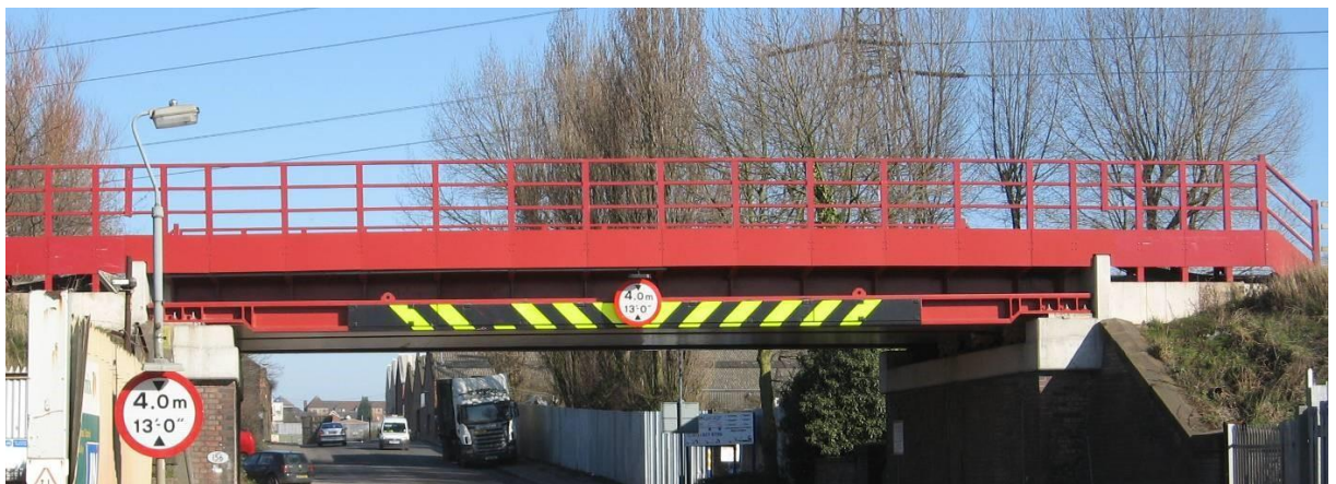
Figure A.5 Collision protection beam to flat soffit bridge supported from abutment Cills
