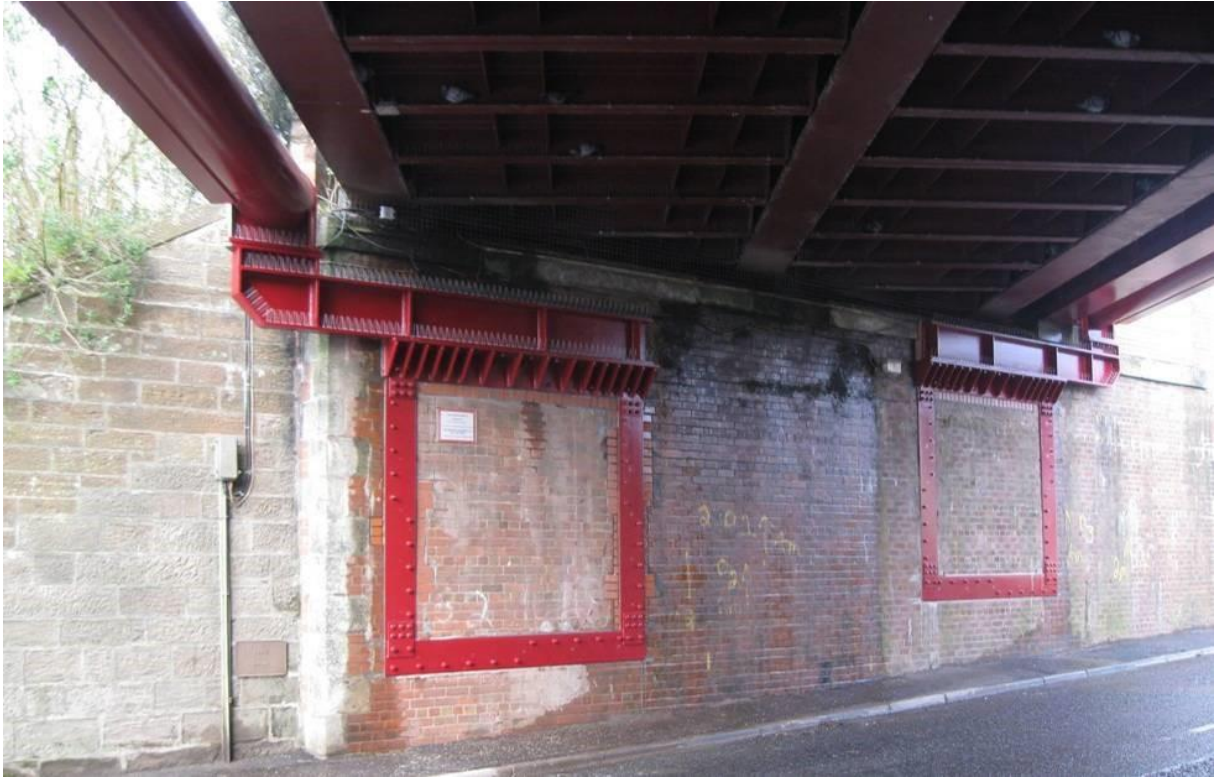
Figure A.2 Collision protection beam abutment supports
