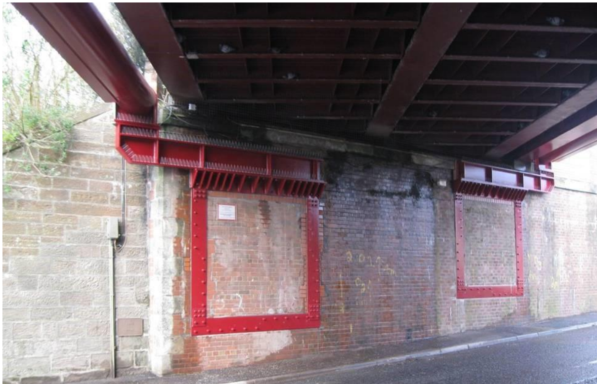
Figure A.2 Collision protection beam abutment supports
