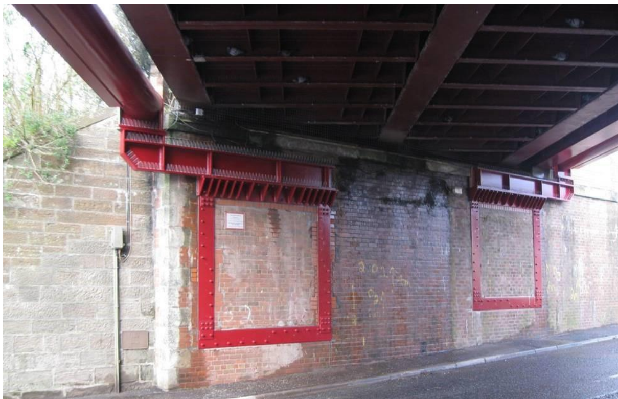
Figure A.2 Collision protection beam abutment supports
