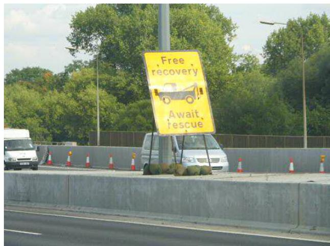
**Figure 3: Sign with 'A' frame located on the top of a concrete barrier**
