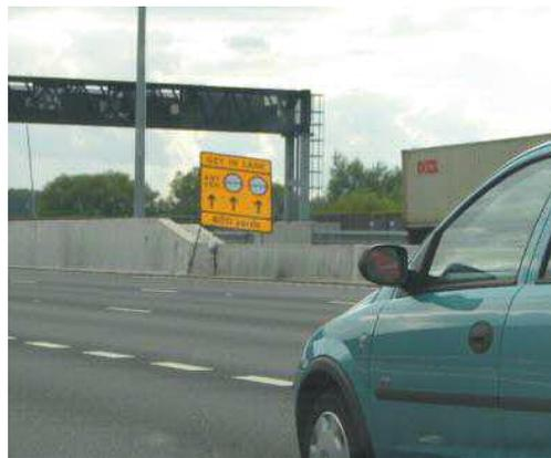
**Figure 2: Sign mounted on an 'A' frame stretched across a concrete safety barrier**
