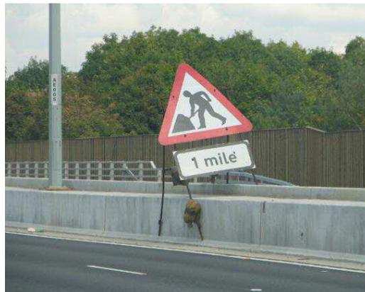
**Figure 1: Conventional 'A' frame in-situ on concrete barrier**
