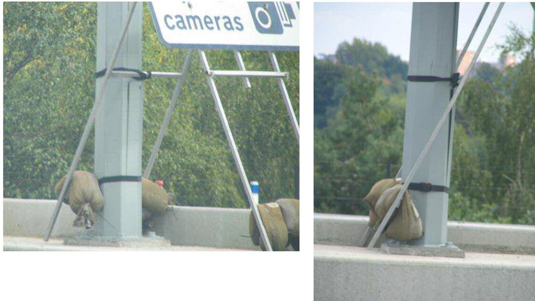
**Figure 4: 'A' frames secured to lamp columns by webbing straps**
