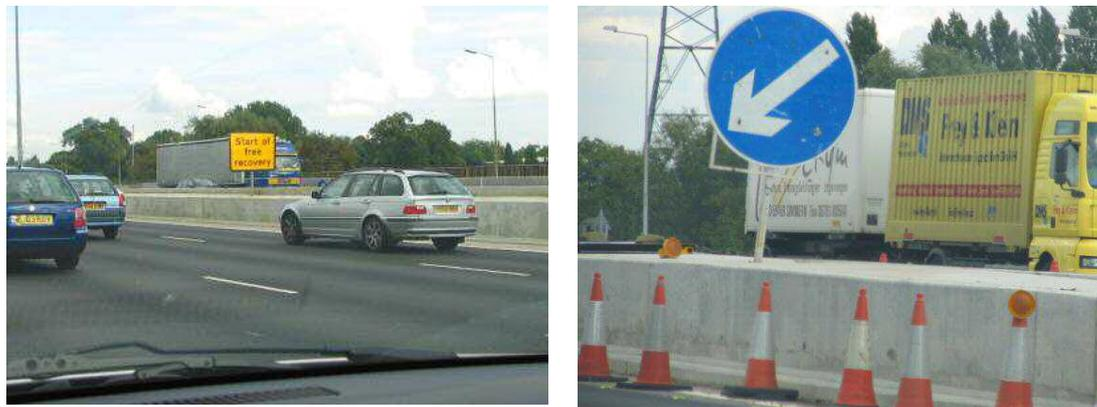
**Figure 5: Temporary traffic management signs mounted on vertical posts in the central reserve**
